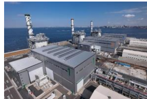
Goi Thermal Power Plants
