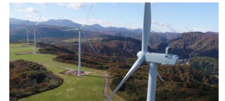
JRE Miyagi Kami Wind Farm
