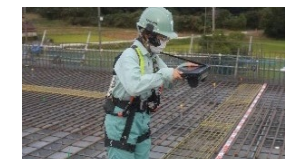
Bar arrangement inspection using AI
