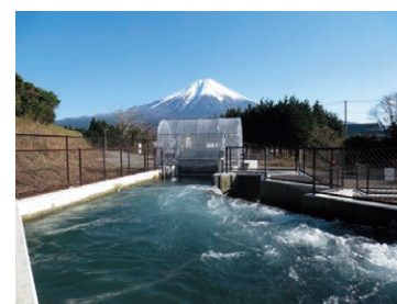
Mibugawa Honmonji First Power Station (Shizuoka, Japan)
