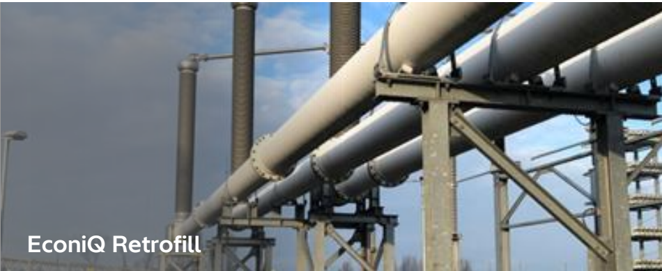
National Grid, UK ELK-3 / 420 kV GI, installed 2016, 755 kg SF6 eliminated
