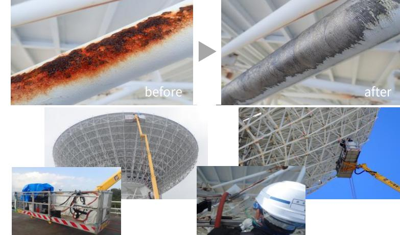
40m-tall parabolic antenna is constantly in motion, temporary scaffolding could not be set up, and the thick rust that is typical of coastal areas could not be removed.
