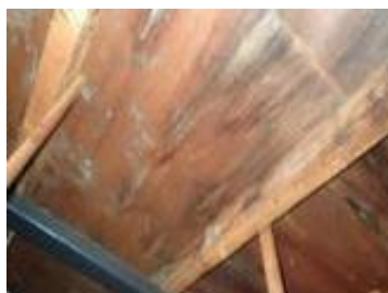
Case in which the roof leaked after sale. A full repair was carried out under the warranty against defects.
