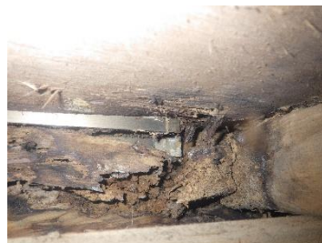
An instance where termite damage was overlooked, resulting in major restoration work including replacement of parts of the wooden structure.
