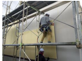
( QD Panel installation )
