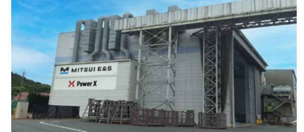
Within the Mitsui E&S Tamano Works site (Tamano City, Okayama Prefecture)
