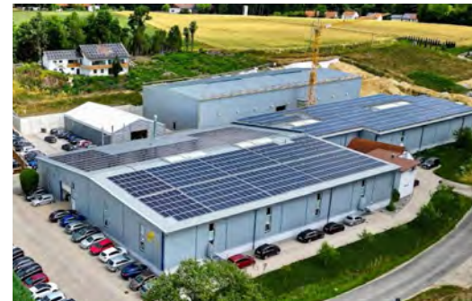
Image of Schmidbauer's facilities in Hebertsfelden, Germany
