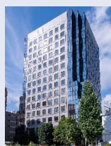
Osaki MT Building
