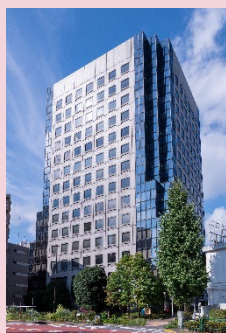
Osaki MT Building
