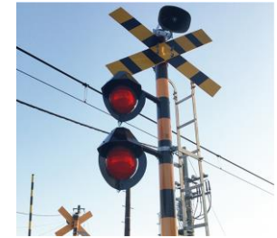
Installing omnidirectional warning lights
