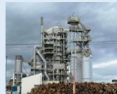
Hachinohe Biomass Power Plant
