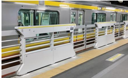
Installing slit-frame automatic platform gates
