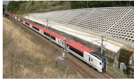
Reinforcing wayside embankments
