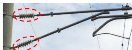
Polymer insulator for overhead wires
