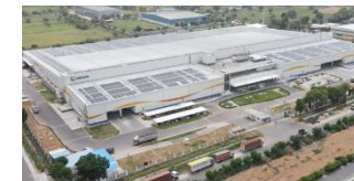
Neemrana Plant in India
