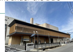
New Waste Incineration Facility for the Aizuwakamatsu Regional Municipal Area Development Association
