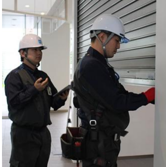
Statutory inspection of fire shutters
