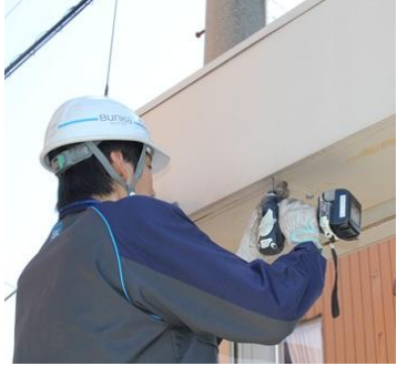
Shutter repair work
