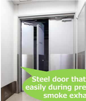
Steel door with an opening-assist Mechanism "Air balancer"
