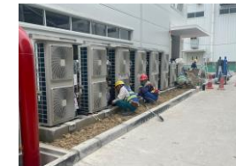
Outdoor unit installation work
