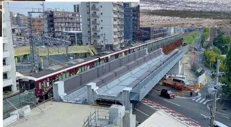
Gt58 manufacturing and erection work as part of FY2025 civil engineering work associated with the continuous grade separation work (Section 5) around Awaji Station on the Kyoto Line/Senri Line Hankyu Corporation (Main contractor) JV of Mori-Gumi Co.,Ltd., SHIMIZU CORPORATION, and Fujita Corporation
