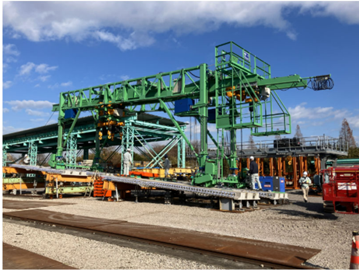
Floor slab replacement machine
