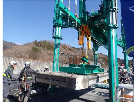
Floor slab replacement works of Nakano Bridge on Chuo Expressway (FY2023) Central Nippon Expressway Company Limited JV of Fuji P.S. and MIYAJI ENGINEERING
