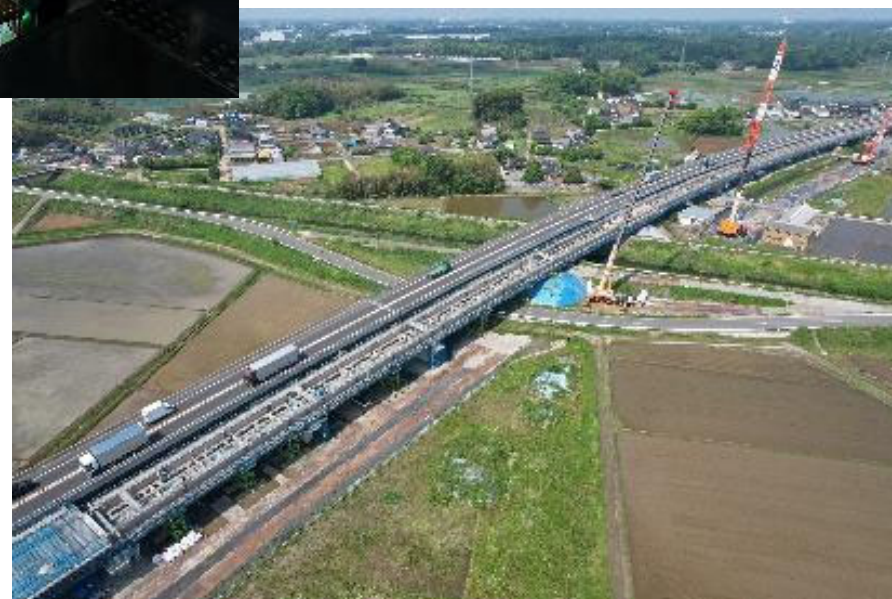
Construction work of the Metropolitan area center communication Expressway Iinuma River Viaduct (steel superstructure) West East Nippon Expressway Company Limited
