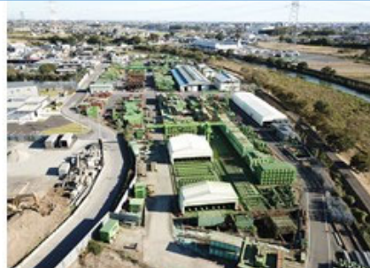
MIYAJI ENGINEERING CO., LTD. Kurihashi Equipment Center
