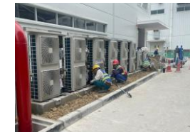
Outdoor unit installation work
