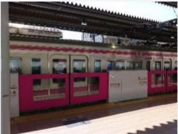
▲ After Platform Door Installation
