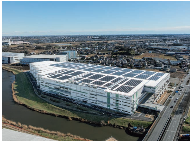
(仮称)LOGI' Q蓮田新築工事
