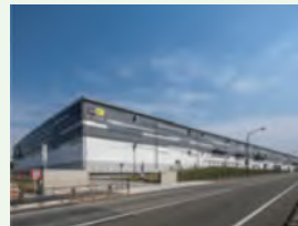
Landport Tama (managed property)
