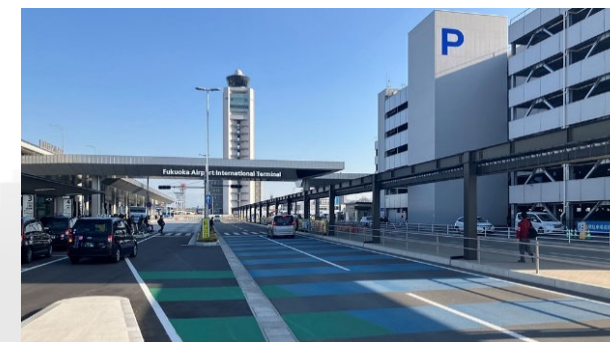
Improvement work at Fukuoka Airport International Terminal curbside
