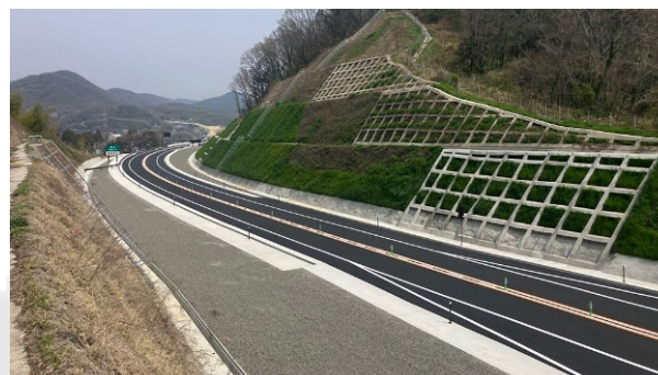
Pavement work on Kasaoka Bypass in Yokoshima area (FY2025)
