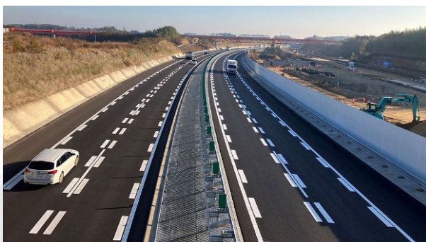
Pavement work on Higashi Kanto Expressway in Narita area
