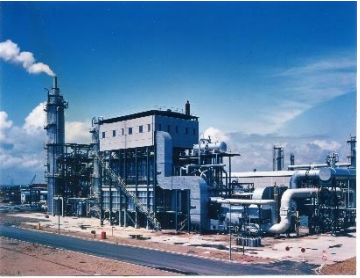
Large-scale hydrogen production facility
