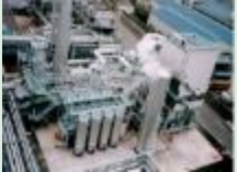
Large-scale hydrogen production facility (Our EPC)
