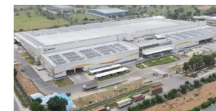
Neemrana Plant in India
