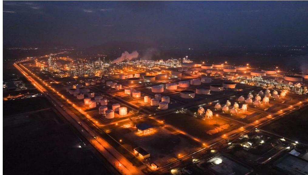
Nghi Son Refinery
