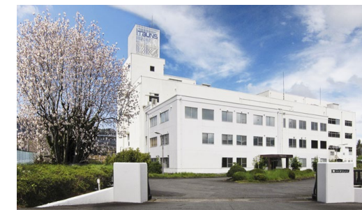
Head Office/Kamishima Factory
