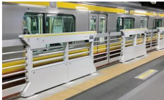
Installing automatic platform gates
