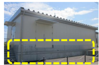
Relocation of electrical equipment to higher places
