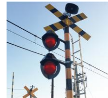
Installing omnidirectional warning lights
