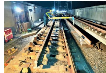
Maintenance work with particular focus (Left: Rail replacement, Right: Signal relay replacement)
