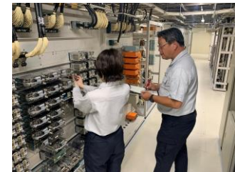
Maintenance work with particular focus (Left: Rail replacement, Right: Signal relay replacement)
