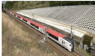
Reinforcing wayside embankments
