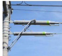
Upgrading overhead wire facilities
